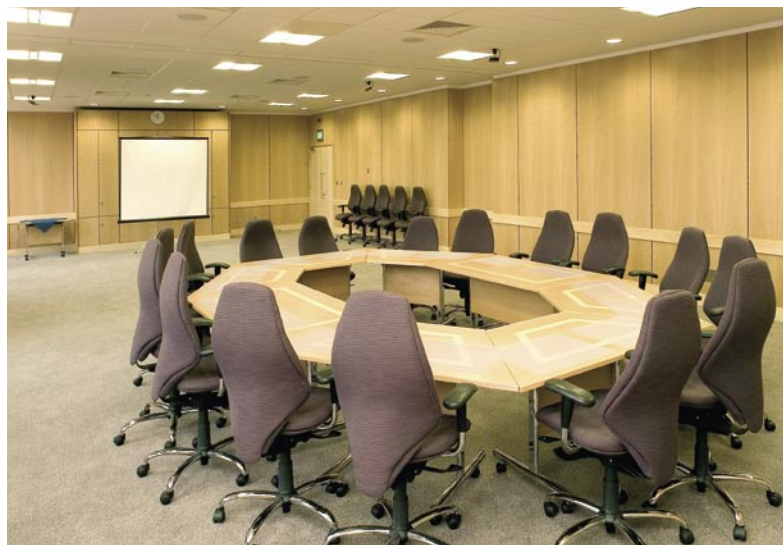
Small systems, such as the boardroom illustrated here, can be programmed and the pre-sets configured via a control panel incorporating programming capability.
